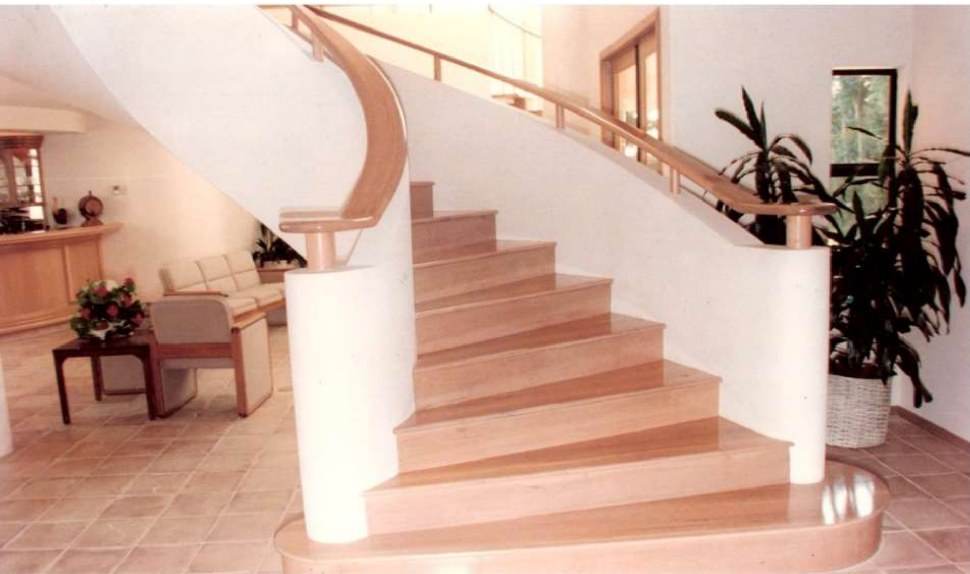
I built this spiral staircase out of plywood and oak. I laid plywood strips up on the curves as a cold-mold similar to the way I built my trimaran.
