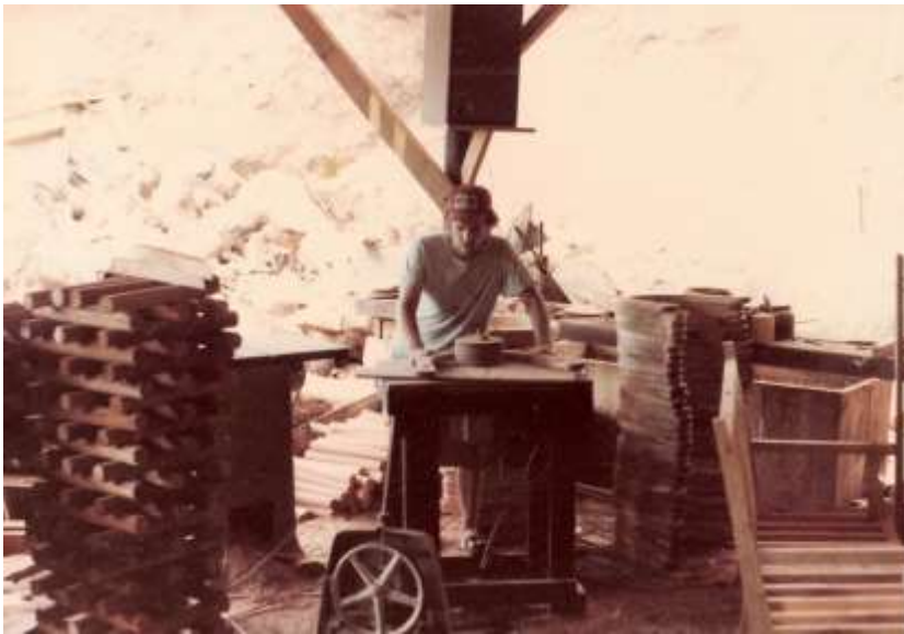
Shaping chair arms on a sanding table that I made.
